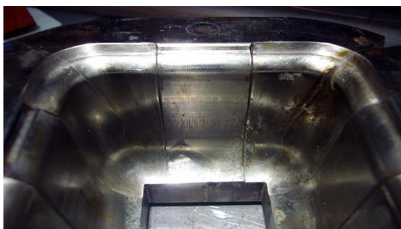
Figure 5. Repair of press-mould dies by filling and welding
